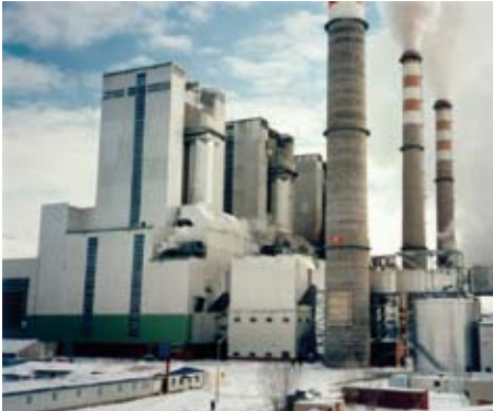
Kagal Power Station with newer unit 3 boiler in the foreground
