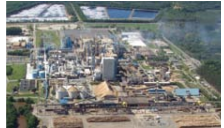
Aracruz Celulose Pulp Mill, Brazil is installed with 260 Clyde Bergemann sootblowers
